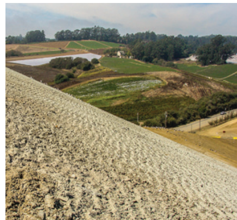
Posi-Shell Intermediate Cover on thin soil leveling layer
